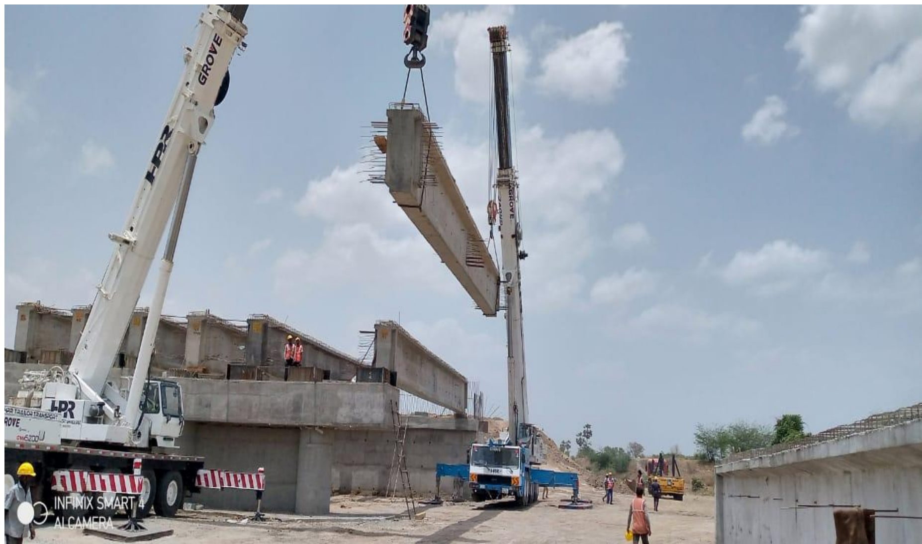
Girder launching at Major Bridge Ch-359+936
