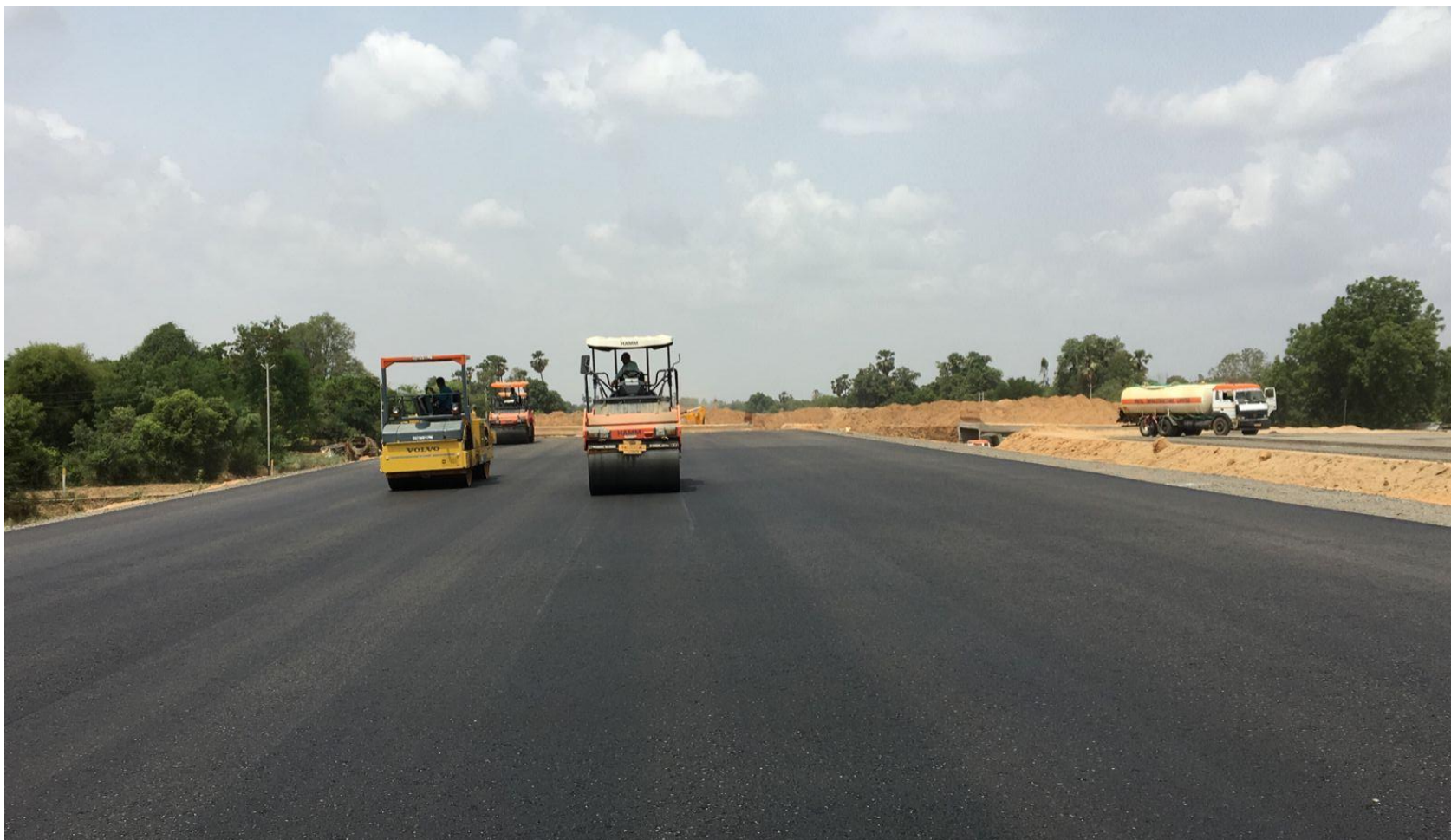
DBM-Ist Rolling In Progress
