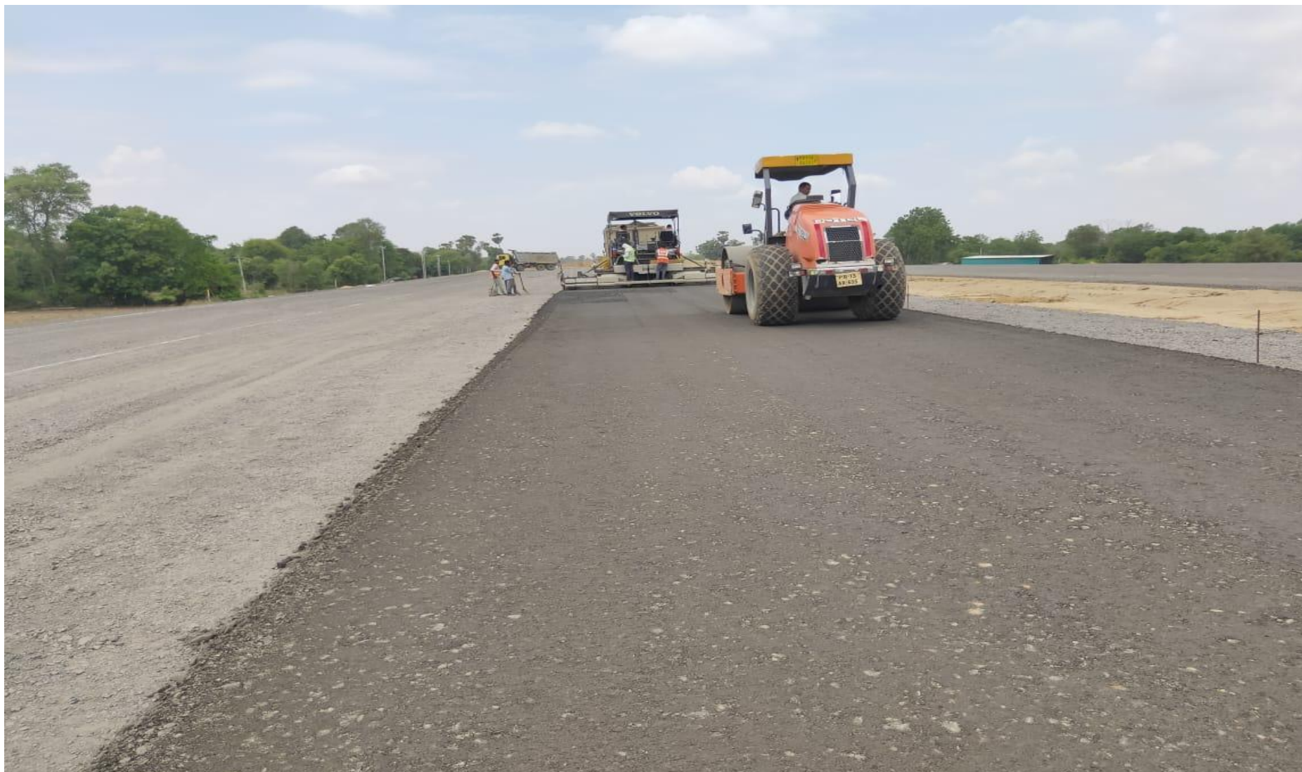
WMM laying in progress
