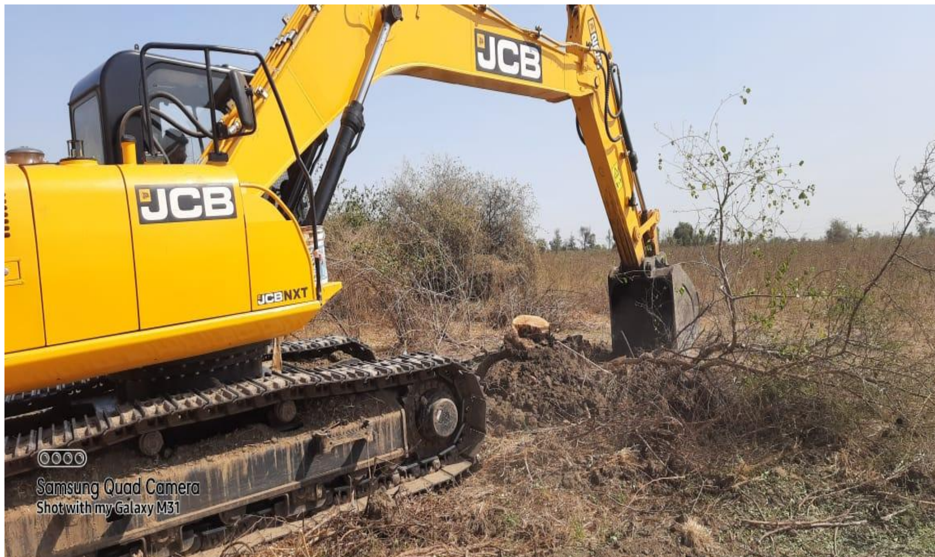
C&G work and Roots removal in progress
