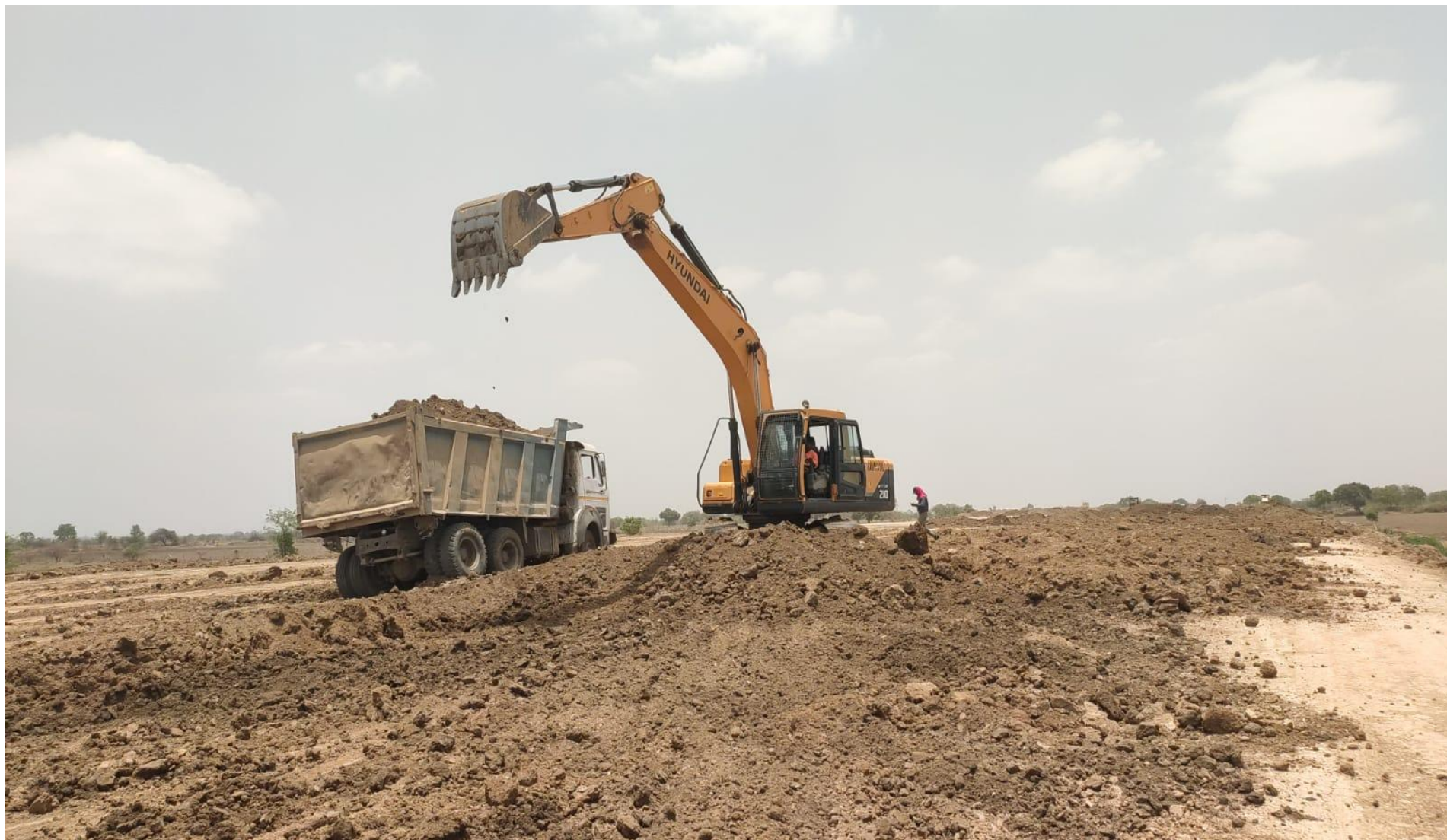
Black cotton soil removing at site
