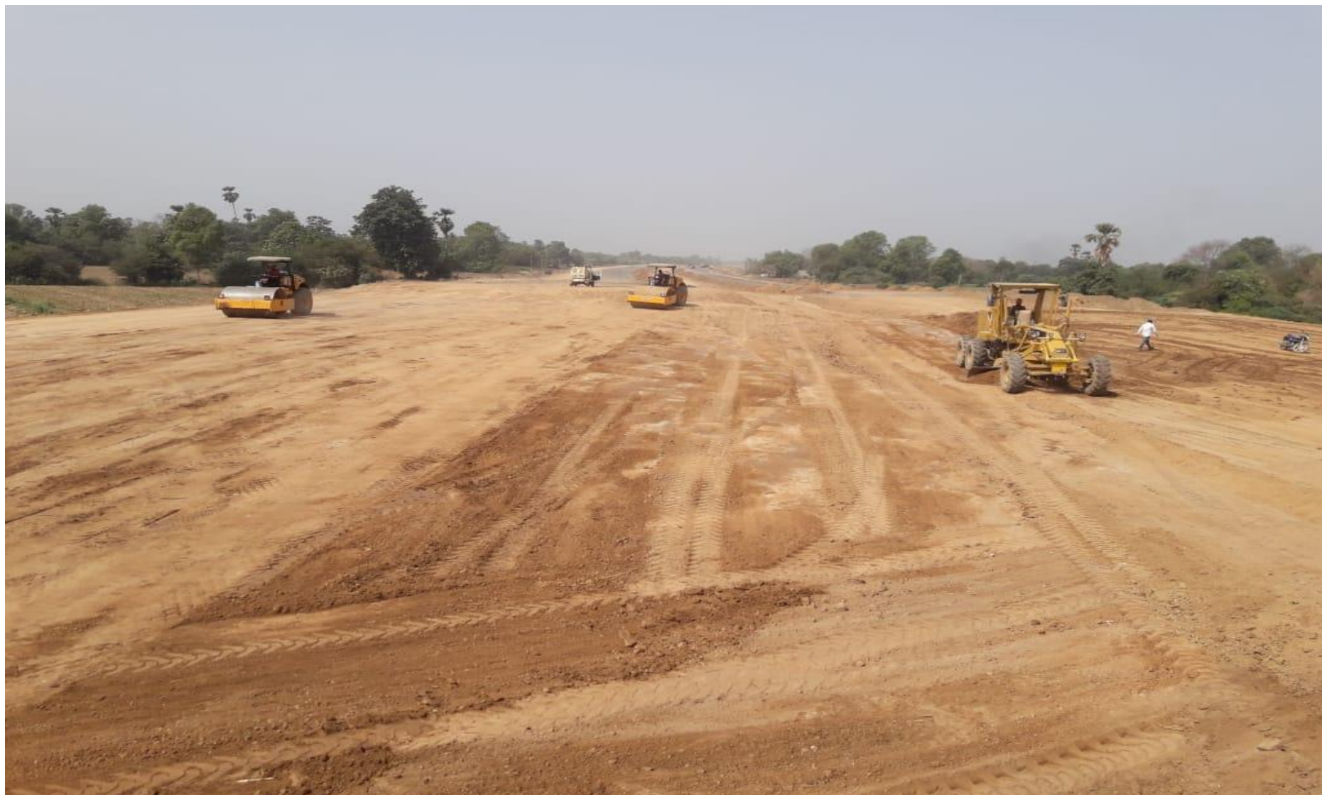
Embankment Layer in progress
