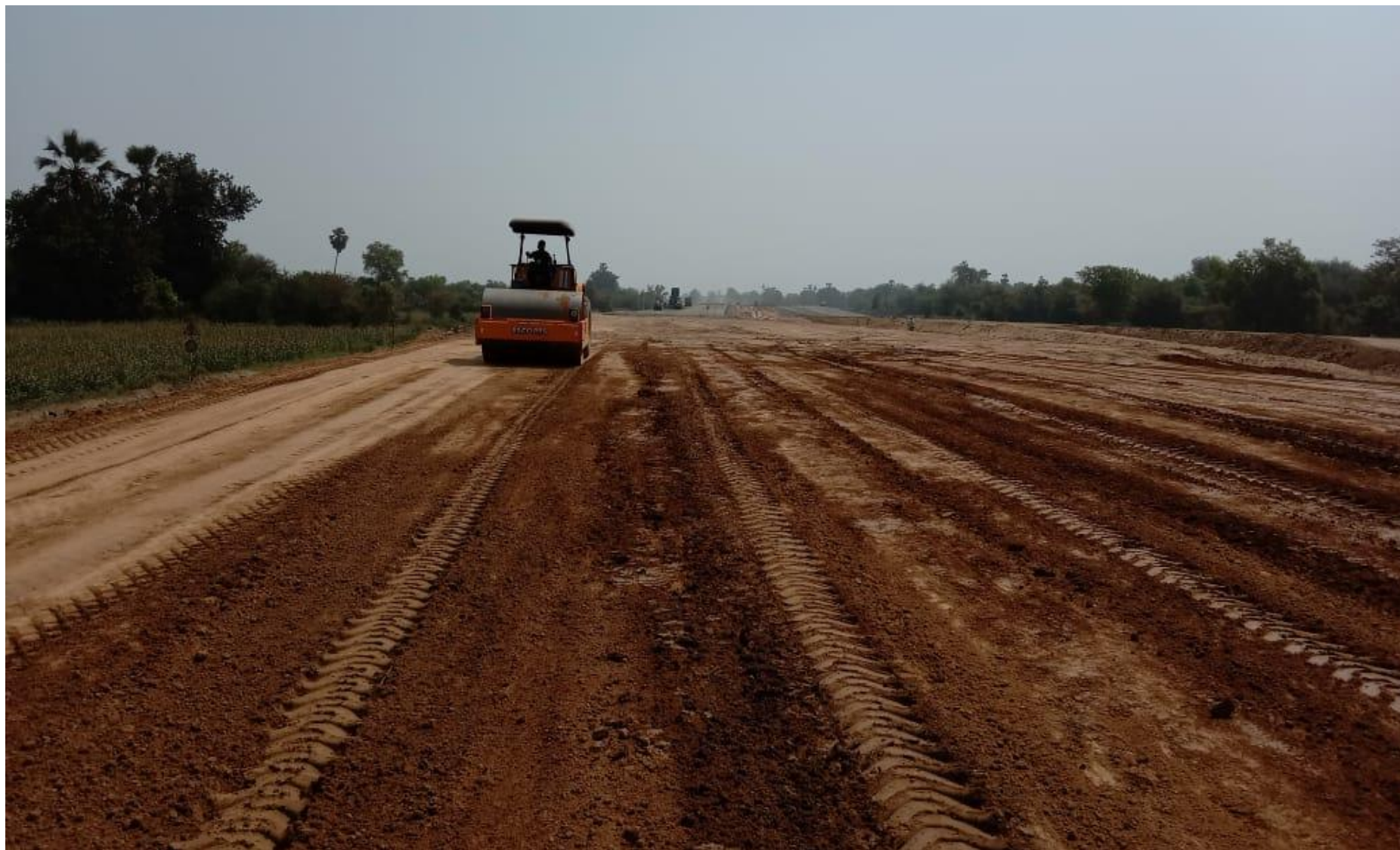
Embankment Layer in progress
