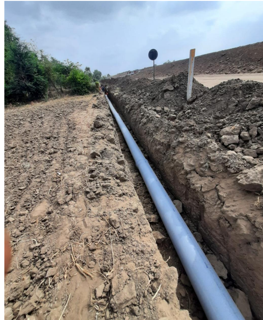
UGPL pipe laying work in progress 356+700 rhs
